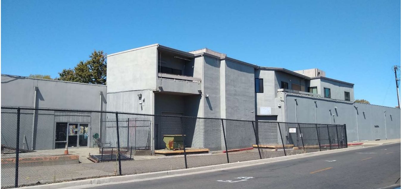
West façade, looking northeast. ESA, 2022.
