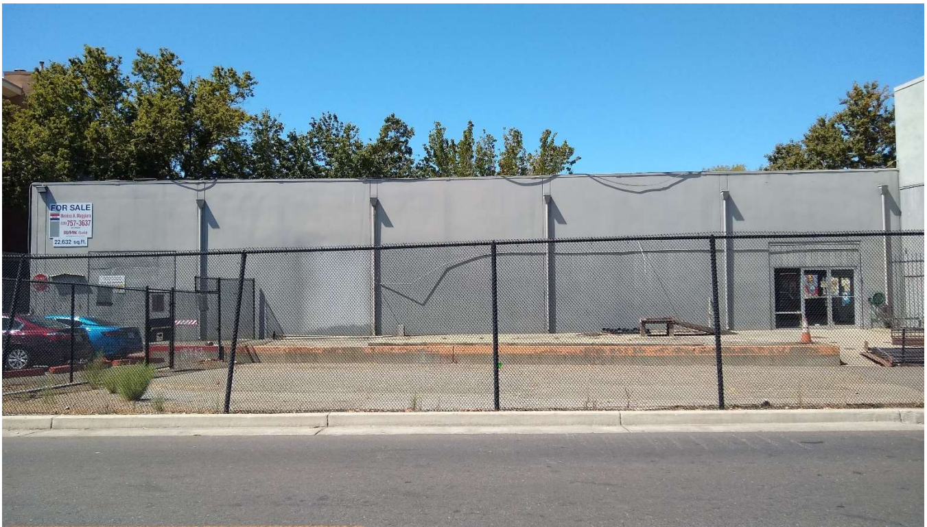
West façade, looking east. ESA, 2022.
